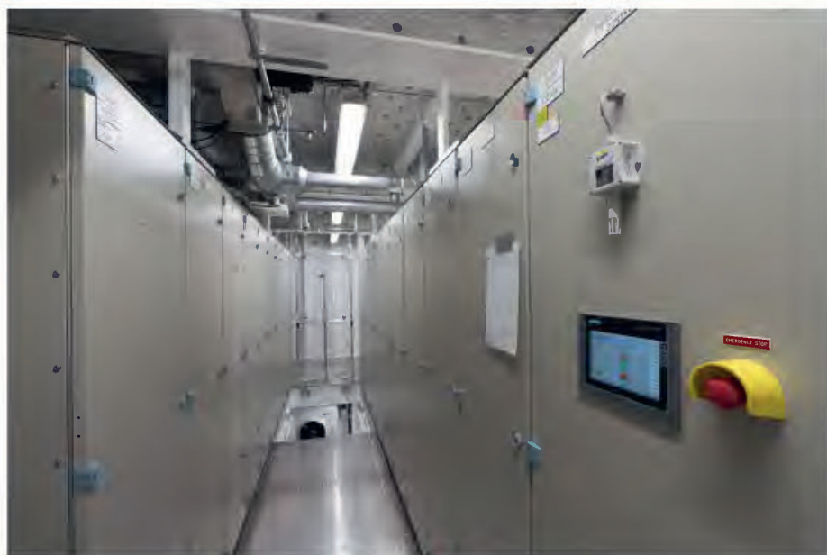
The battery cabinets in the lower hull.
