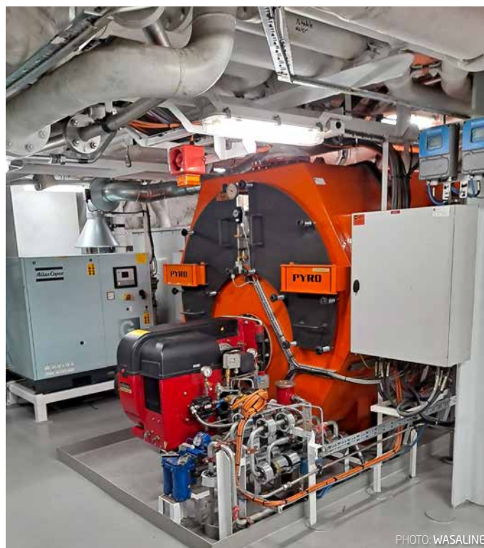
A Pyro auxiliary boiler.
