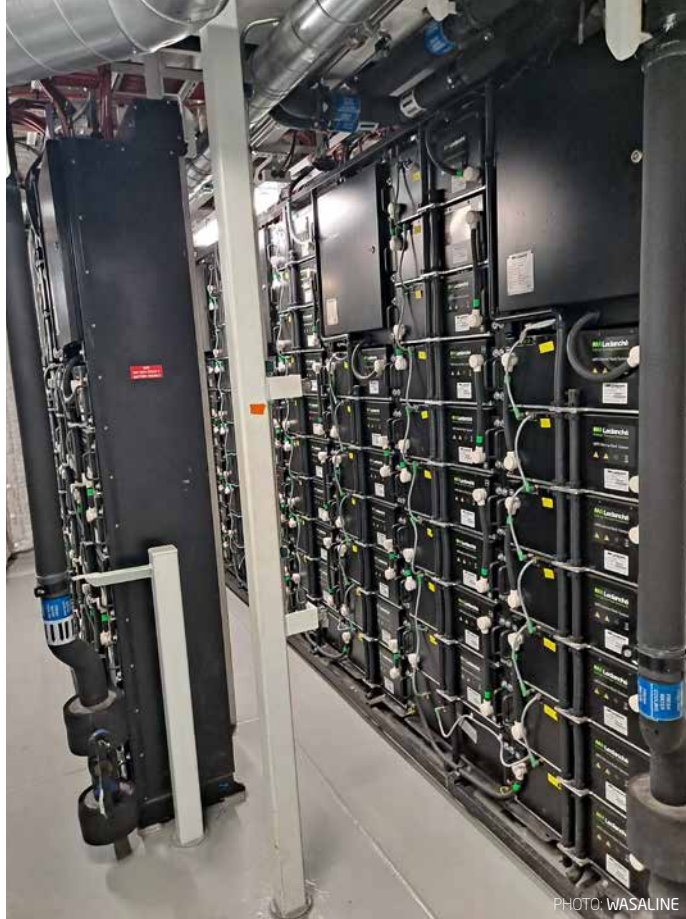
The Leclanche battery rack system.
